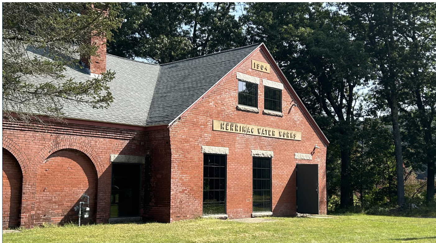
A view of the Merrimac Water Works Building
