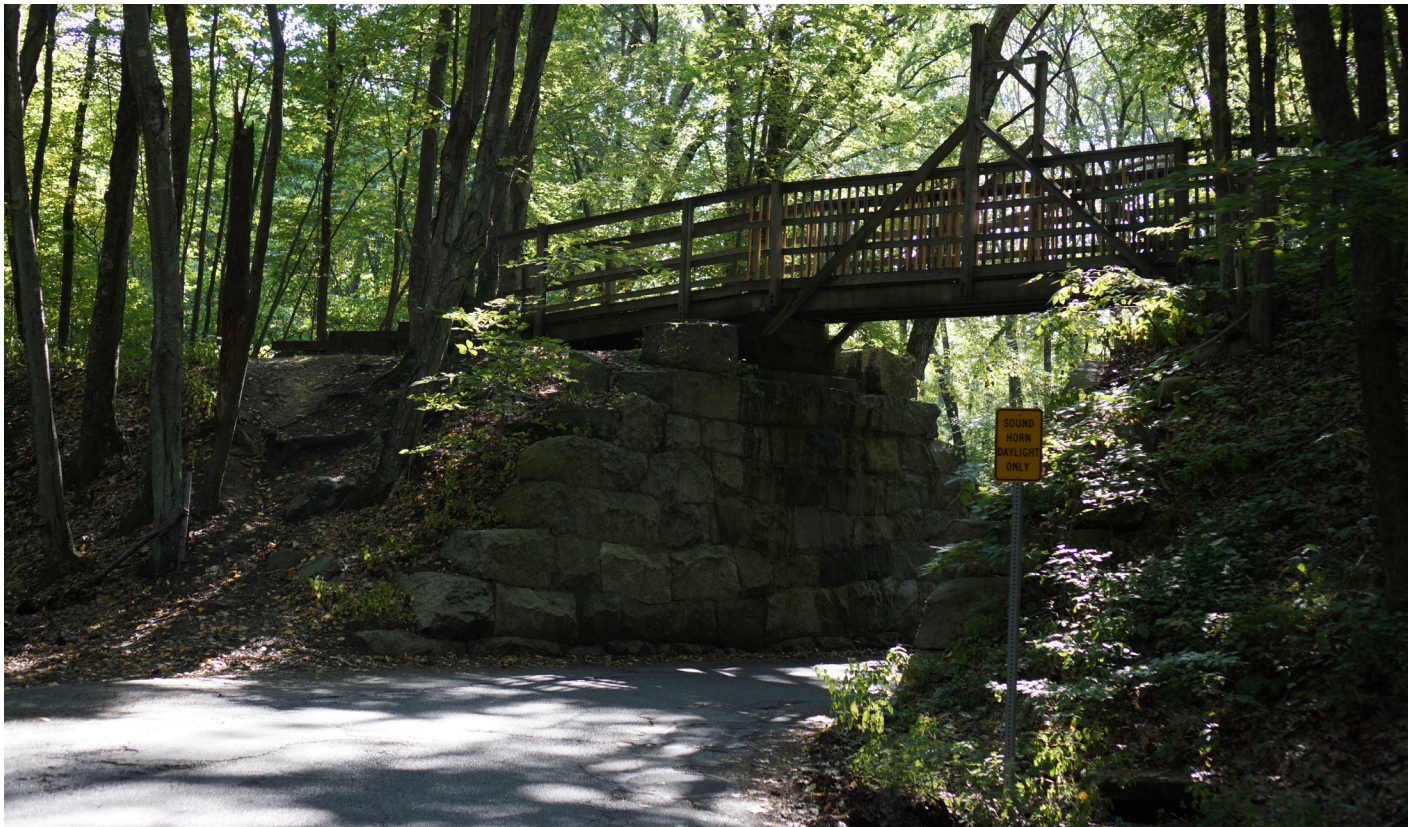
A view of the Jay McLaren Trail Footbridge
